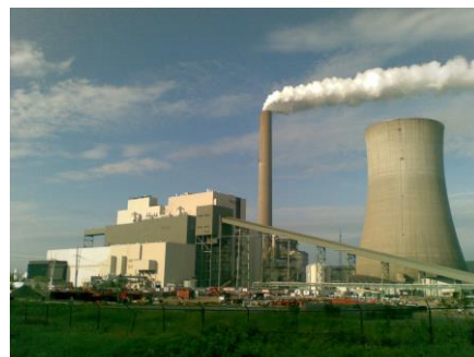
Trimble County Generating Station
